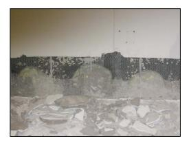
The original plan was to demolish the lower portion of the walls in the areas where the insulation was missing, install insulation, and repair the interior finishes. This plan included an extended period where closing the main section of the museum would be required. The photo to the left shows a small test area where the plaster was removed, as in the original plan, to confirm the effectiveness of the approach.
