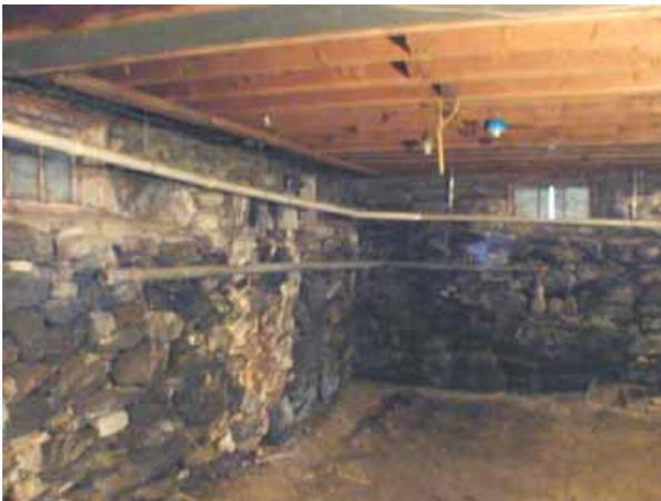
Before: Classic dry-laid stone foundation with signs of frost damage.
