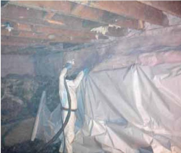
The top of the wall is insulated; then, the A/V barrier is suspended from the SPF just above the high-water level to complete the envelope and provide a drainage outlet for seasonal water infiltration.
